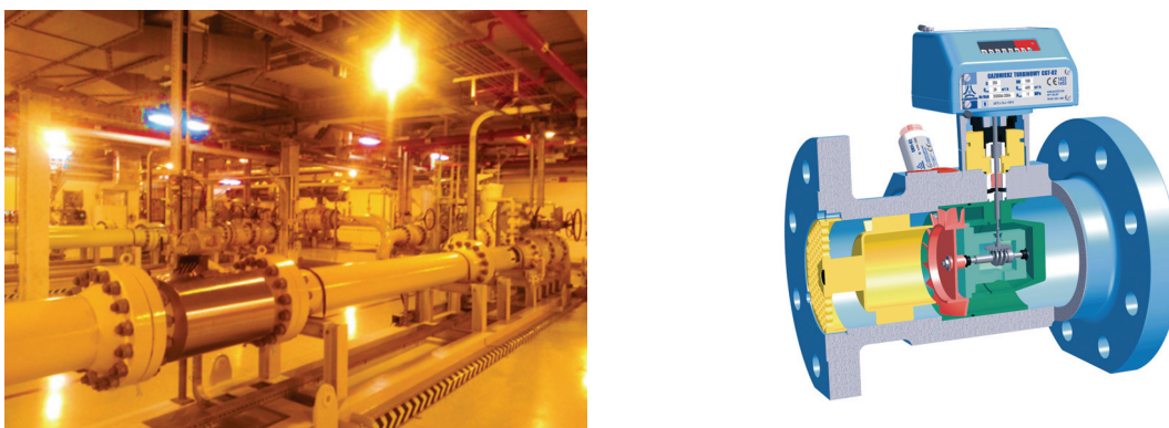
Fig. 2. Left: gas metering station at the LNG terminal in Świnoujście, Right: typical turbine gas meter (COMMON S.A.)
