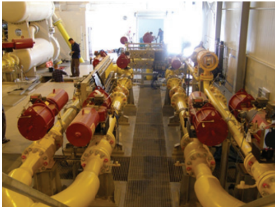
Fig. 5. High pressure gas meter calibration facility built by GAZ-SYSTEM SA. CS – compressor station, SV – shut-off valves, FCV – regulating valves, MUT – meter under test, WS – working standards, TS – transfer standards
